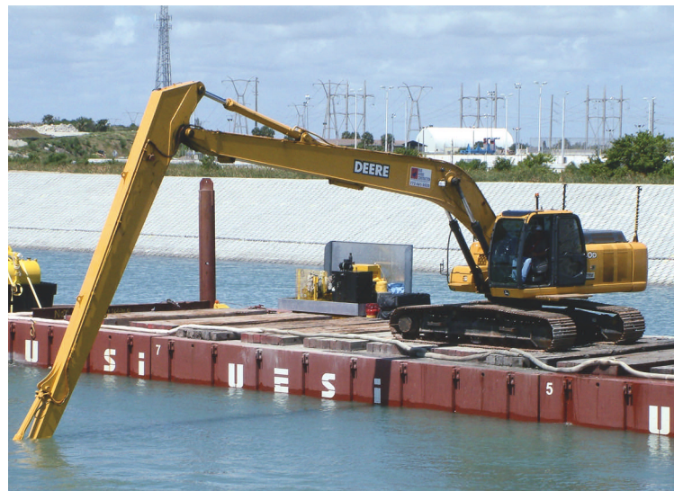
Waterproof position sensors on the boom, stick and bucket track their motions and integrate with GPS positioning so excavators can grade the canal floor 25 feet under the surface.
